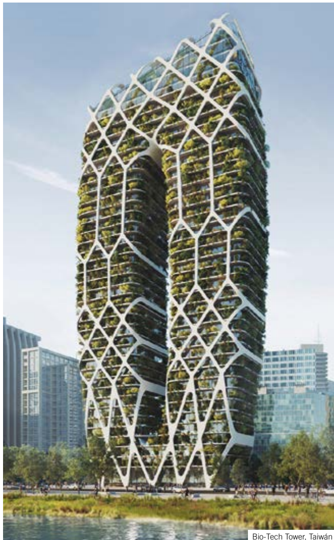
Bio-Tech Tower, Taiwán
